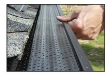
2. Screw front edge of panel to top of gutter lip using pre-set fastening points. Take care not to over-tighten the screw.
