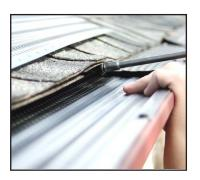
4. Outside Corners - Cut first panel on 45 angle. Cut second on 45 angle, leaving a slight overlap through which you can secure mitered panels together.
