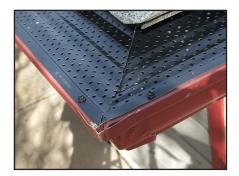
Gutter Guard is an integral part of a well functioning Rain Water Collection system.
